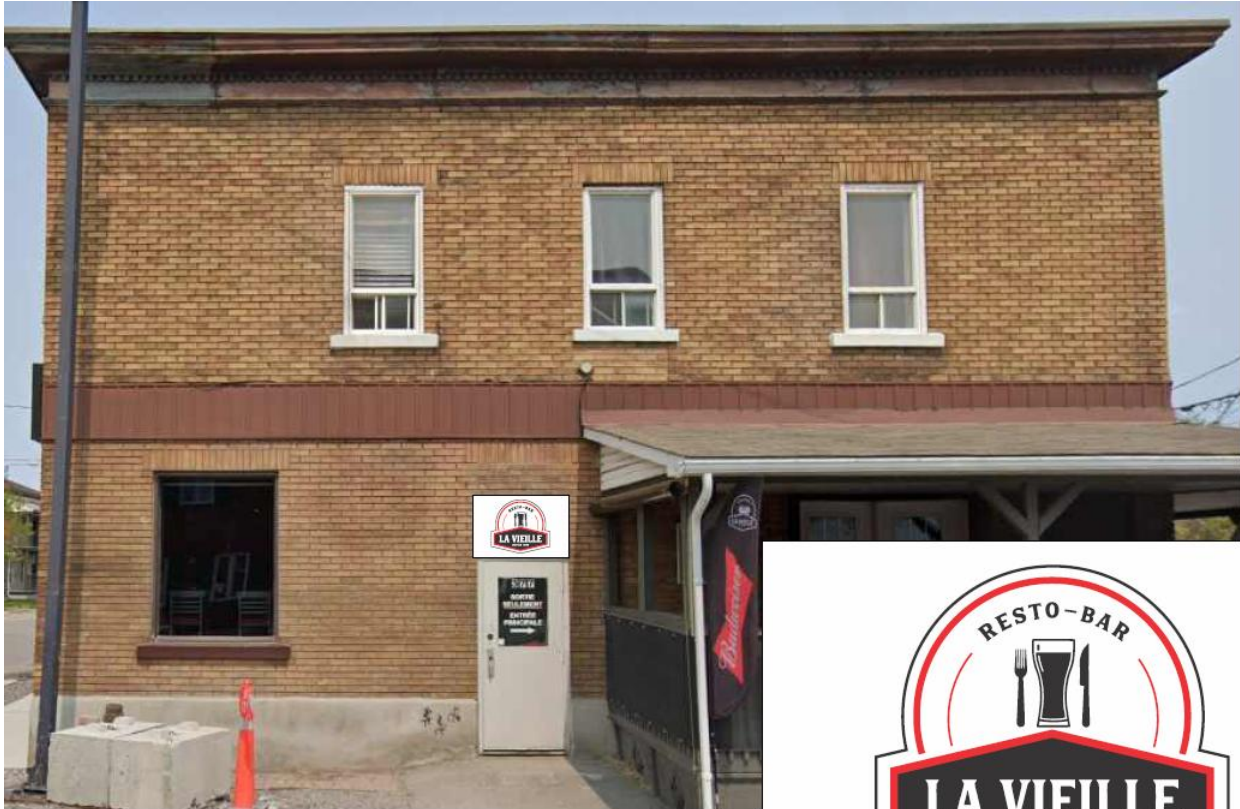
Non illuminated alupanel sign, 1/8" thick fix on the brick wall
